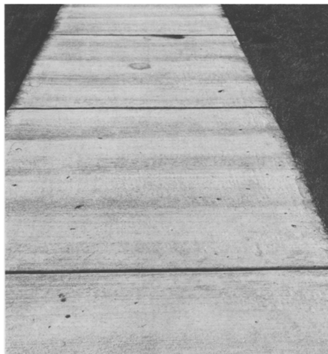
FIG. 2. Photograph of uncoated NRRL sidewalk showing many popouts. Circular area at top is a plug where core was removed for compressive strength measurement.
